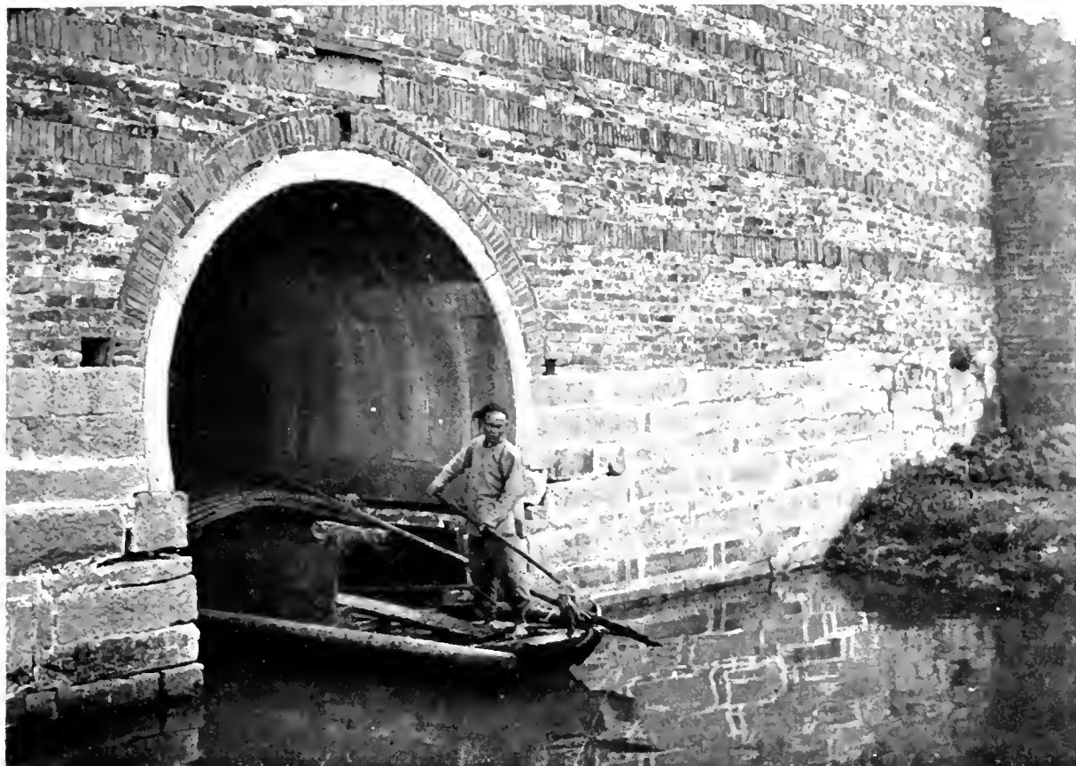
SUCHOW: ONE OF THE WATER GATES
